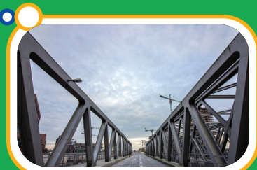
Structures for roads & bridges
