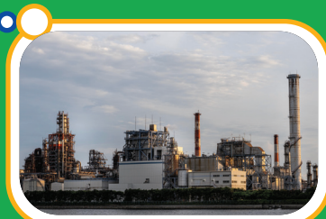
Primary & secondary structures for boilers & turbine generators
